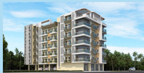
PROJECT NAME : Sai Niwas LOCATION : Income Tax, Patna PROJECT COST : 12.00 cr BUA IN SQFT : 40647
